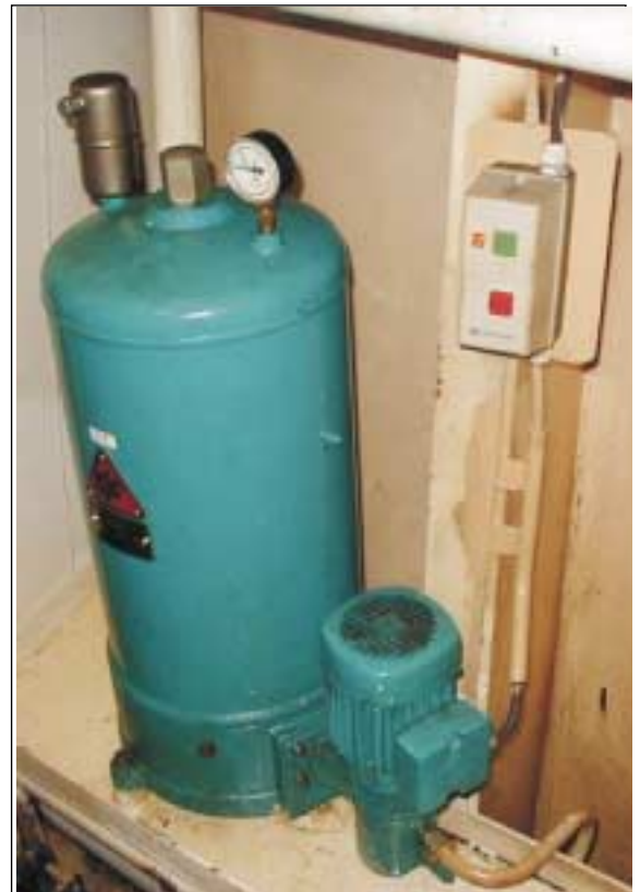
CJC™ Fine Filter type HDU 27/54 MZ installed on the reduction gear of M/S Chilean Reefer.
