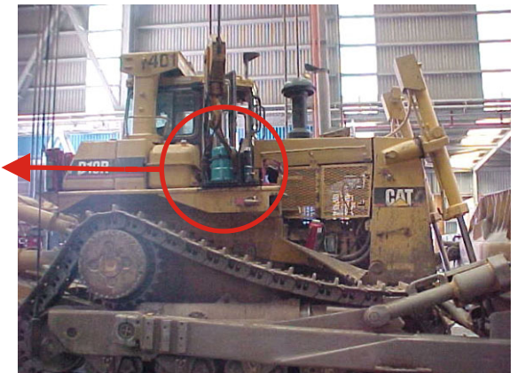
The installation of CJC™ Filter
