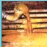
Water Contaminated Oil
