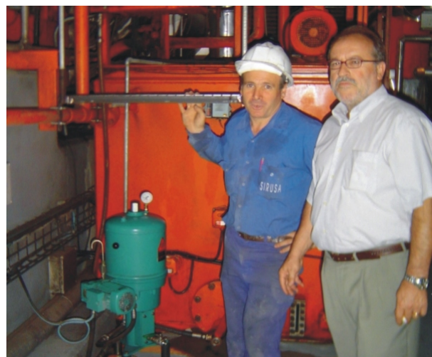
Installation of the CJC™ FineFilter PTU2 27/27
