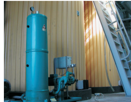
For depth filtering of hot-oil plants, a new type CJC™ Fine Filter is developed, which can resist the high pressure in the system. The model is an HP 27/108 and is presently in operation at Daloon, filtering two huge boilers, each containing approx. 7,000 litres of hot-oil.
